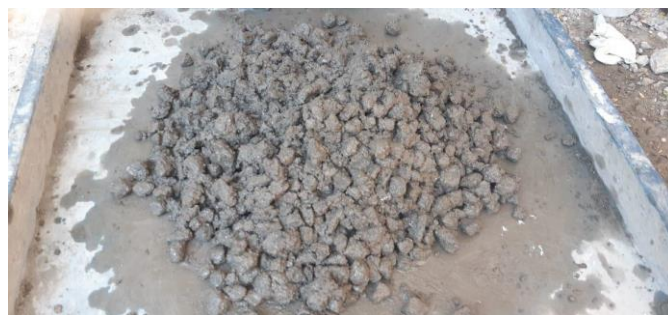
Fig-5: Mixing of luminescent concrete.
