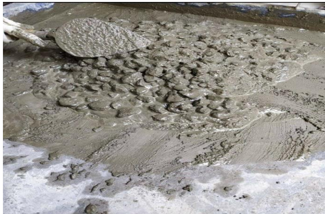
Fig -1: Mixing of conventional concrete.
