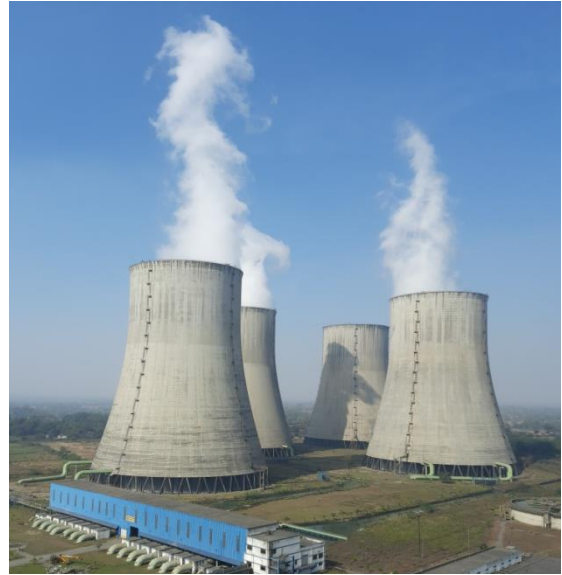
Figure 1 - Counter flow NDCT
