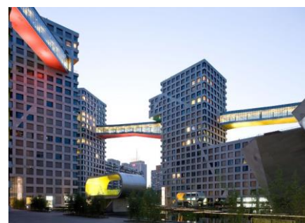
Fig -3: Sky Bridge
