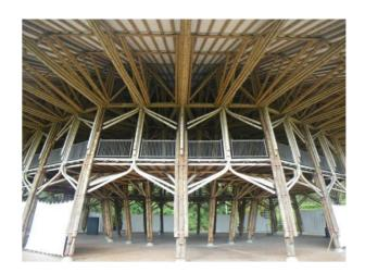
An application of triangular method is displayed within the structure which is situated in an earthquake prone area within the Andes. Simón Velez, the architect behind this structure has made use of sunshine materials in triangular alignment. (Photo by: Ross Stein)
