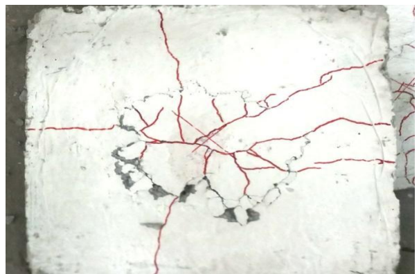
Figure-13: Crack Pattern of M-1
