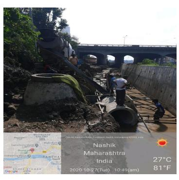
A. Cause of position of man hole with site condition. The man hole for an pipe laying work should be 30 mts as standerd but due to site condition it may varies in length than the standard length given.
