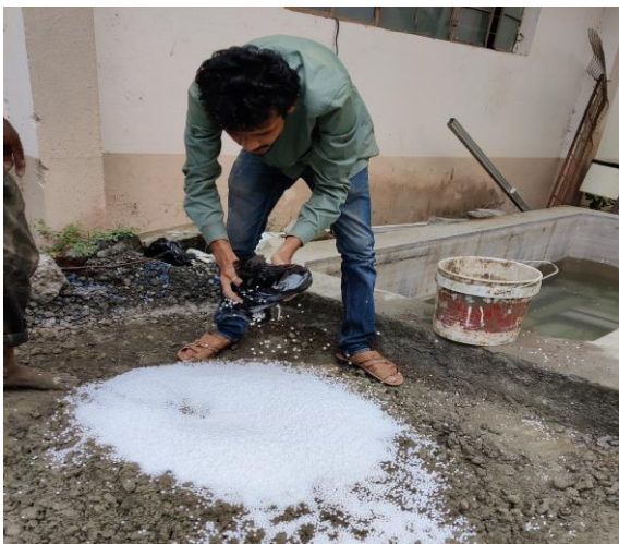
Fig-1. Mixing of EPS BEADS in concrete
