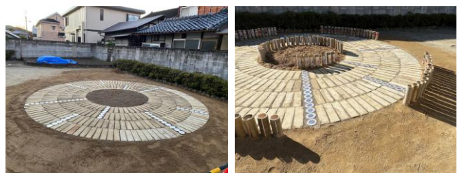
Fig -12: Square paved with bamboo fiber block.
