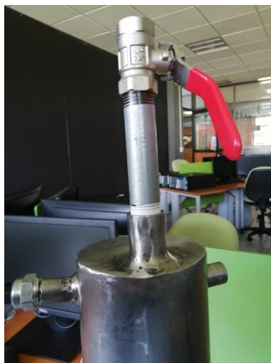
Fig- 3 Placement of relief valve.
