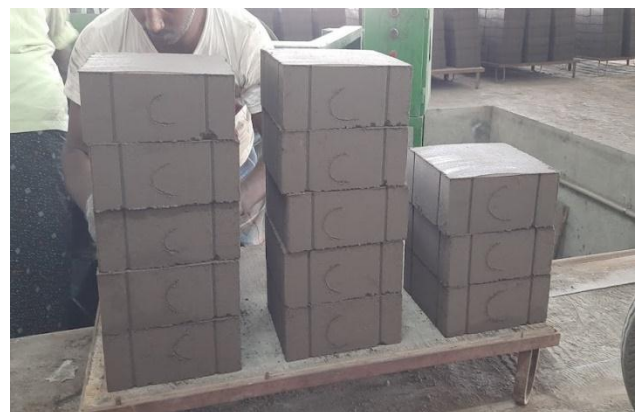
Figure 1 Casting of solid blocks
