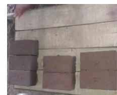
Fig 4.1 Casting of brick
