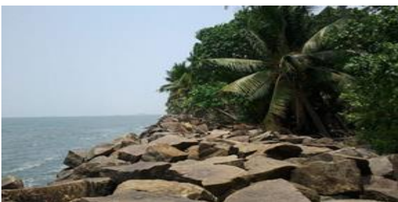
Figure 17: Temporary remedies using seawalls. (Retrieved from https://india.mongabay.com/2018/06/keralas-climate-refugees-increase-as-the-sea-eats-into-the-coast/ )
