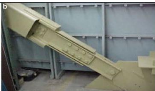
Figure-03: Friction Damper
