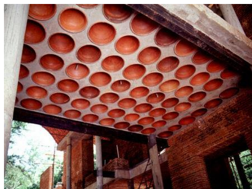
Fig-9: filler roof slabs
