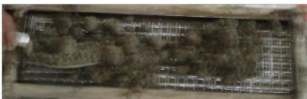
(a) Placing the mortar on mesh
