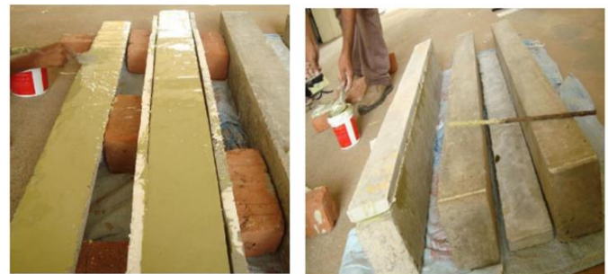
Figure-4 Application of epoxy resin on beam and Strengthened beam
