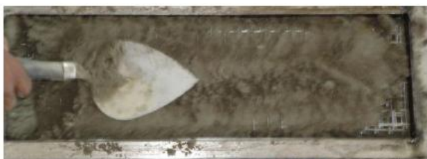
(b) Spreading the mortar on mesh
