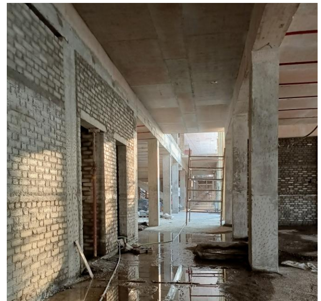
Image no:-2 Conventional Construction Work
