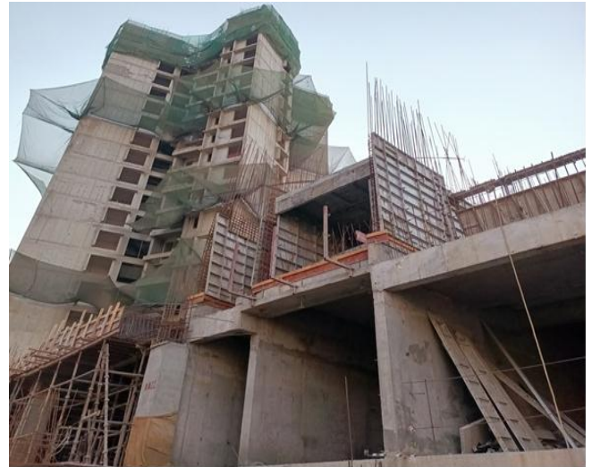
Image no:-1 MIVAN formwork Construction
