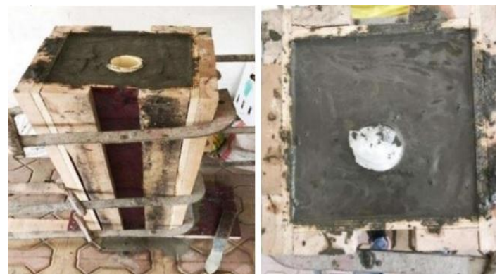
Fig -3: Column casting with CPVC and HDPE pipe
