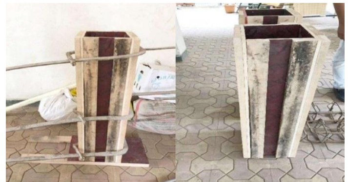
Fig -2: Column formwork
