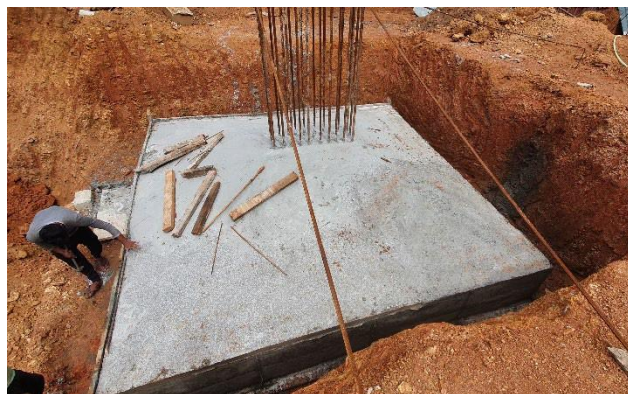
Figure 7: Completed RCC work
