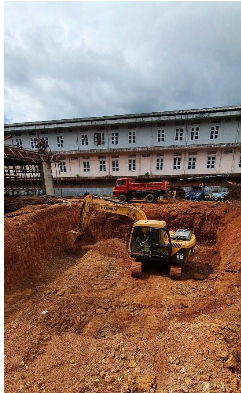
Figure 4: Land excavation using excavating machine
