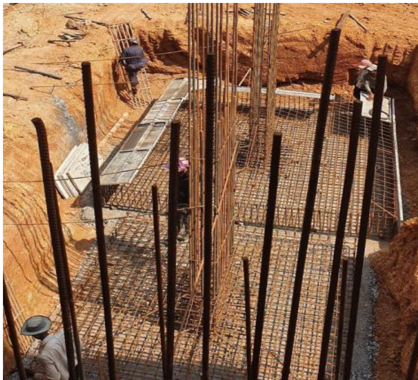
Figure 6: Laying reinforcement bars
