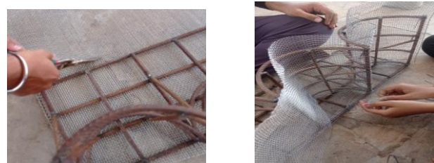
Image 2- Fixing of bars and meshes
