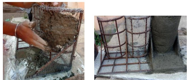
Image 3- Application of mortar
