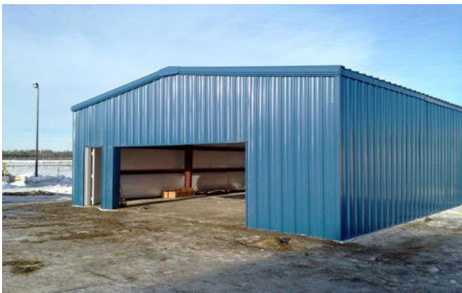
Fig -1: Steel façade frame after cladding
