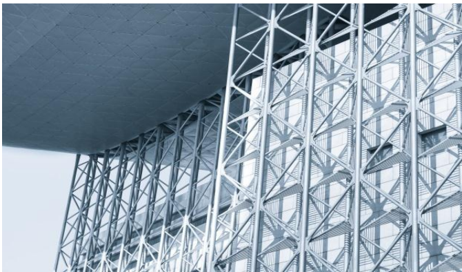
Fig -1: Steel façade frame before cladding
