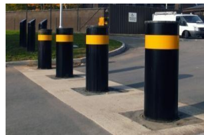
Fig -10: Road blockers
