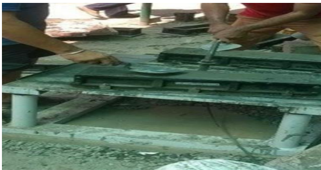
Fig.1: Beam moulds on vibrating table
