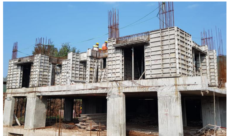
Fig-1: D Building 1 st Floor Shuttering
