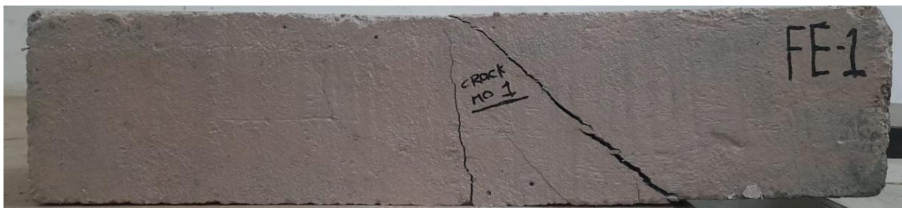
Fig -12: Cracks developed on longitudinal section of FE- 1
