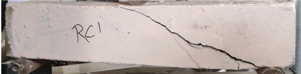
Fig -3: Cracks developed on longitudinal section of RC- 1
