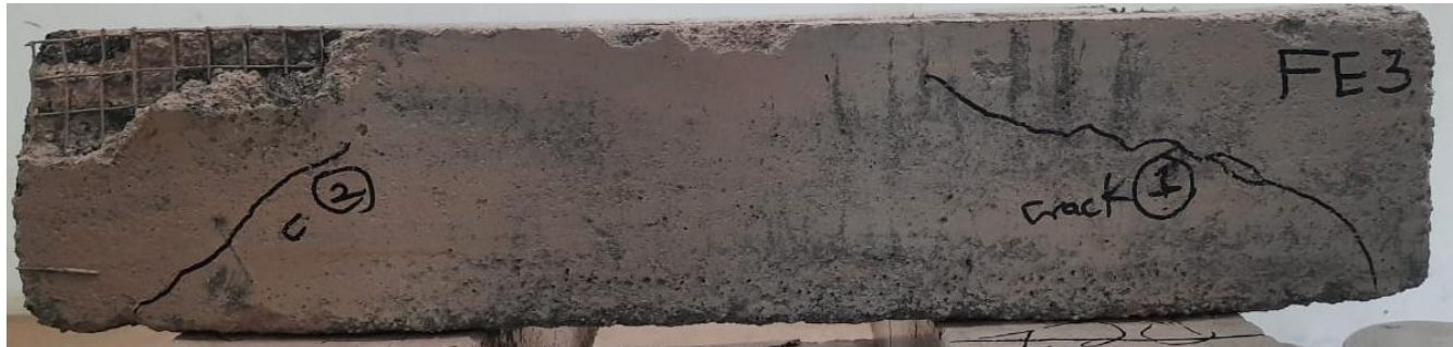
Fig -18: Cracks developed on longitudinal section of FE- 3
