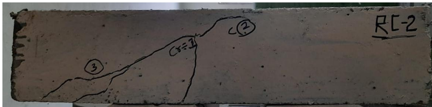
Fig -6: Cracks developed on longitudinal section of RC- 2
