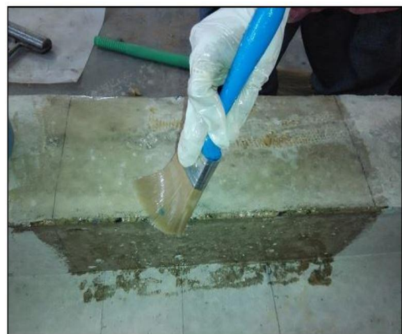
Fig 3: Application of epoxy and hardener on the beam
