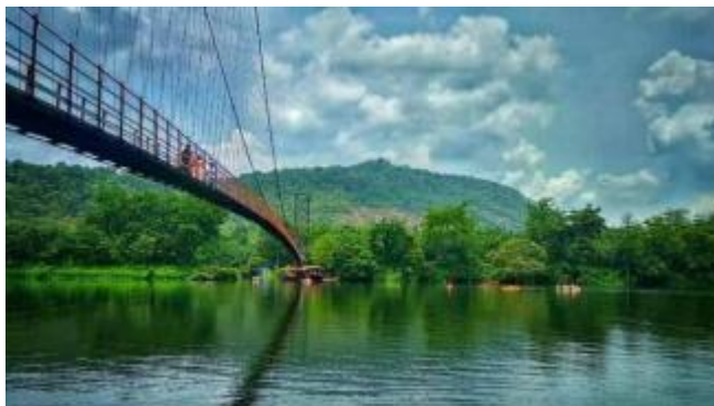
Fig - 2: Inchathotty Suspension Bridge
