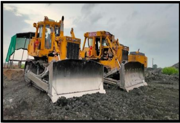
Fig6. Levelling of uneven land using coal soil
