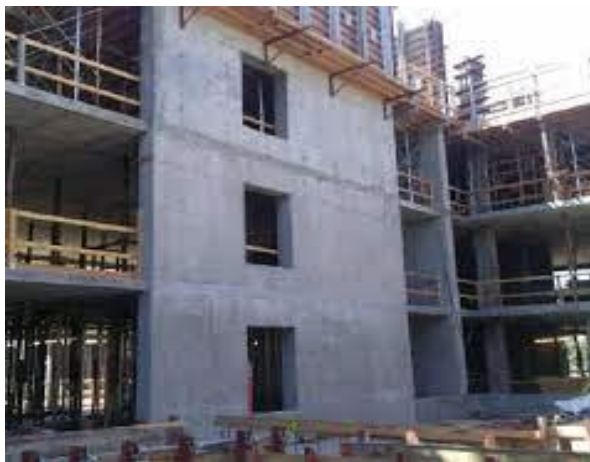
Fig-2 opening in shear wall
