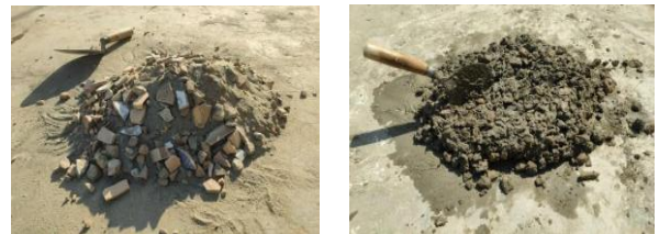
Fig.6- Mixing of Material
